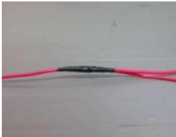
Figure 8 - Isolate the connection
